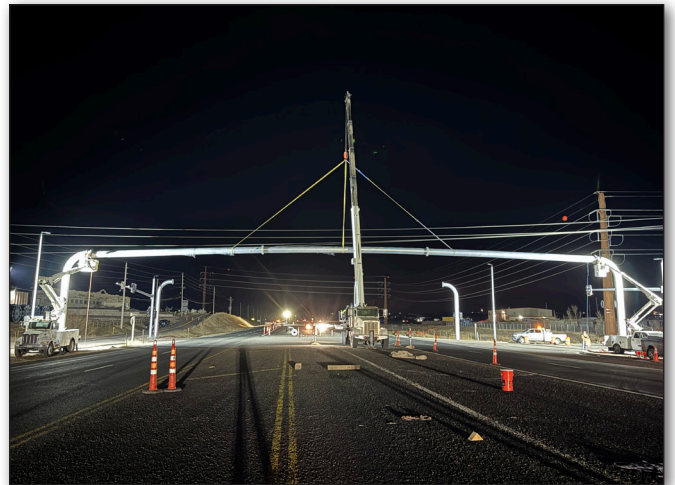
Figure 2 US Highway 85 Traffic Signal
